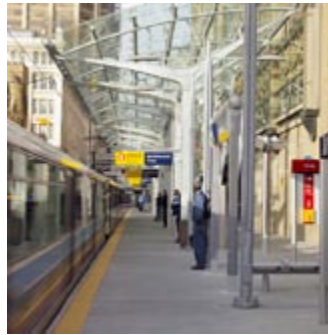
7 Avenue LRT Refurbishment | photo: Robert Lernermeier
